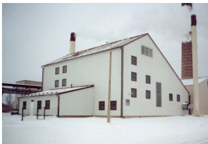
Boiler house in Ludza Latgale Region
